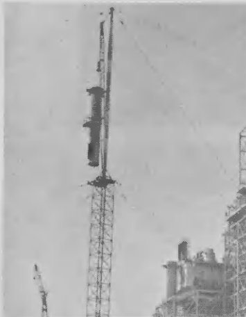
One major lift is handled by the 307-ft. derrick crane: a section of the PCAR smokestack. In about half an hour of skilled maneuvers, upward and downward, the section came down safely on the ground.
